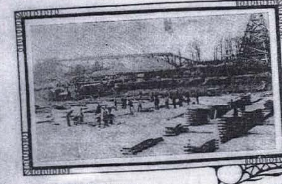
FLOOR OF A FILTER BED. Down Under the Earth Broad Expanse of Concrete Will Be Foundation for the Bed That It to Make Pure the Water Furnished Washington.
