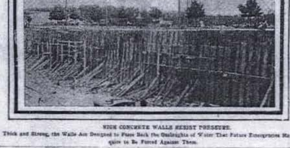
THICK CONCRETE WALLS RESIST PRESSURE. Thick and Strong, the Walls Are Designed to Resist the Onslaughts of Water the Future Emergency May Bring to Be Faced Against Them.
